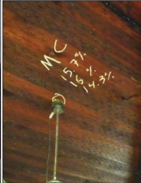
Figure 6 Glulam deck on bridge 1360
