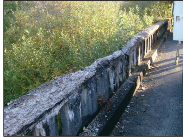
Figure 2 Sylvia Creek Guardrail
