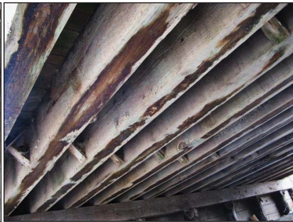
Figure 8 Sawn timber stringers on Summers Lane Bridge
