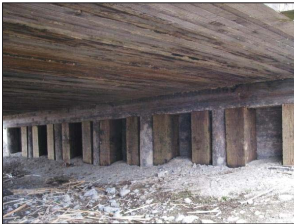
Figure 7 Longitudinal slab deck on Old Midland Rd. bridge
