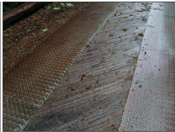
Figure 10 Steel running plates and transverse timber deck on Knopki Creek Bridge
